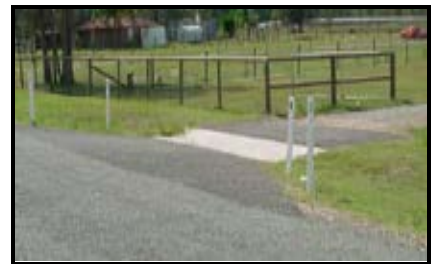
CONCRETE INVERT ACCESS
