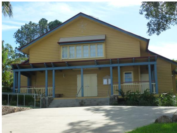
Zamia Theatre, Tamboorine Mountain (Local Heritage Place)
