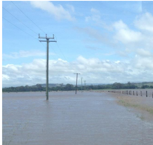
Figure 1: Flooding at Wilsons Plains Road, Harrisville, 2013.
