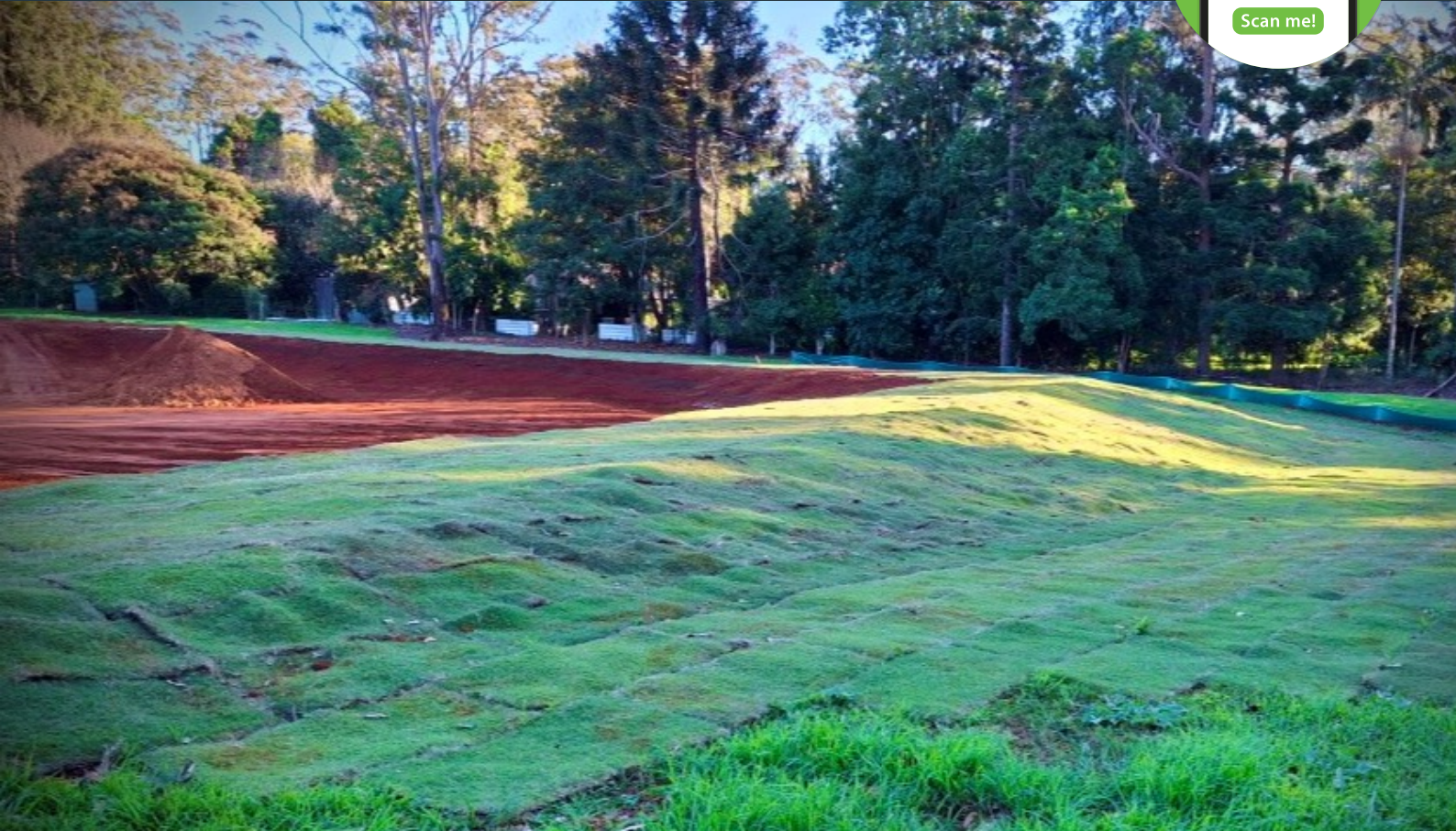
Image of the Detention Basin Construction - June 2025 Walk Precinct
