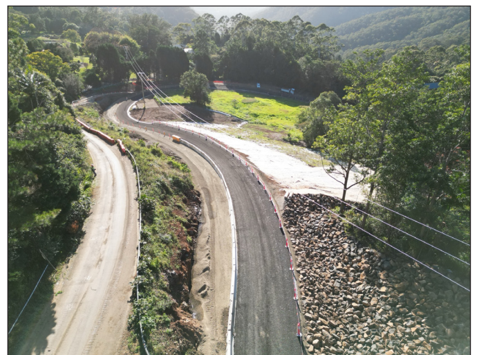
Image 2: The newly constructed road alignment
