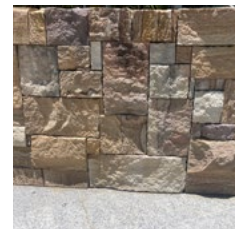
Figure 4: Example of regular stone pavers
